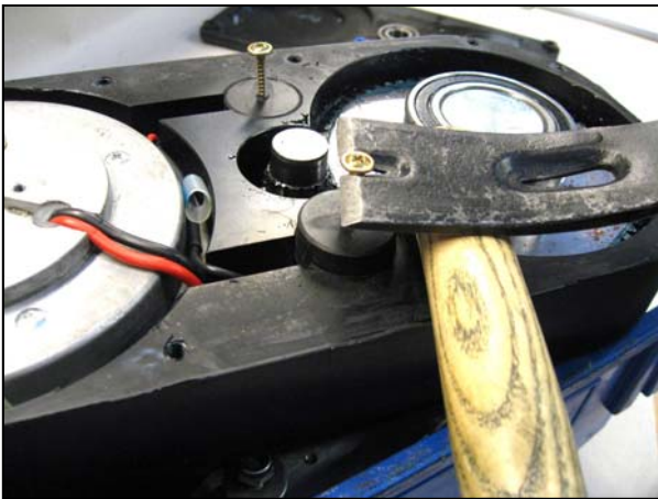
Use a crowbar to pull out the POM blocks. Watch out that you don't damage the drive.
